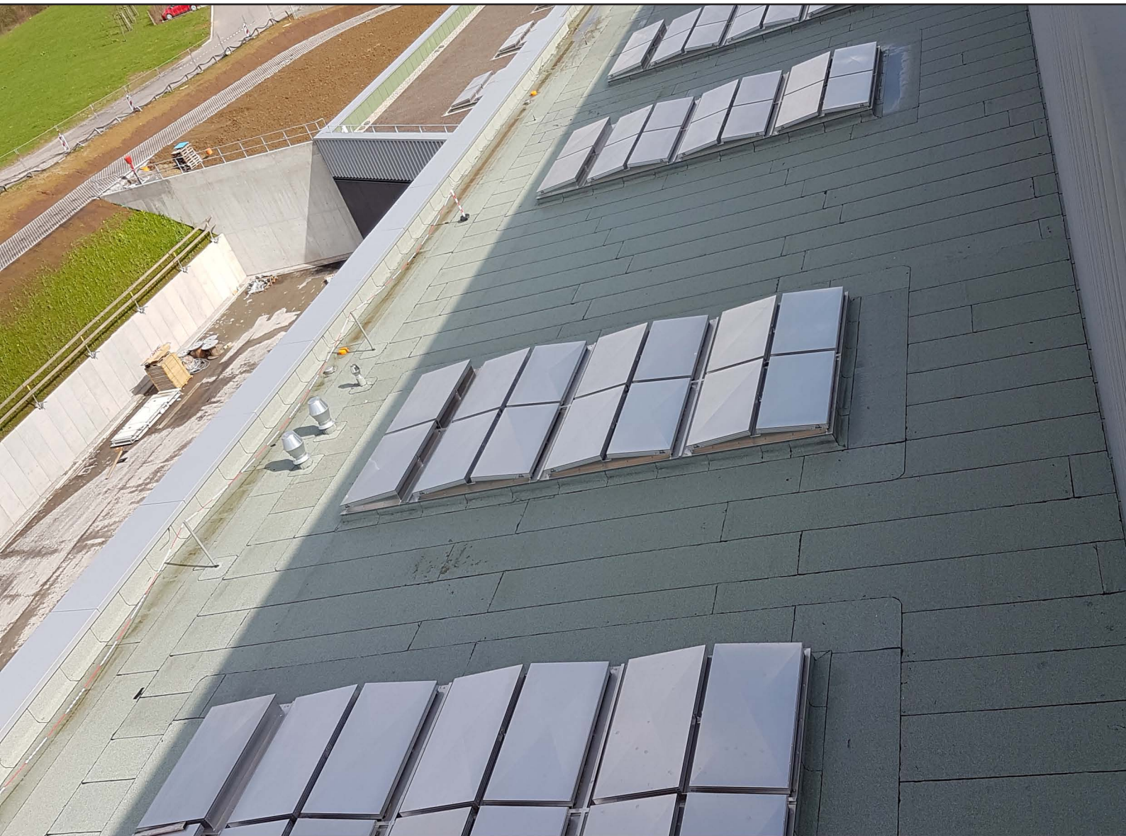
Big picture: SafetyHatch pressure relief flaps with aluminium opening panels
